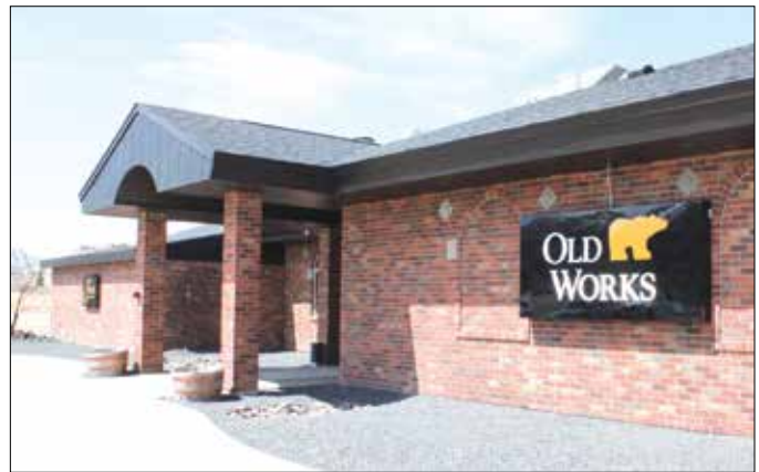
The Old Works Golf Course's clubhouse has been newly remodeled.
